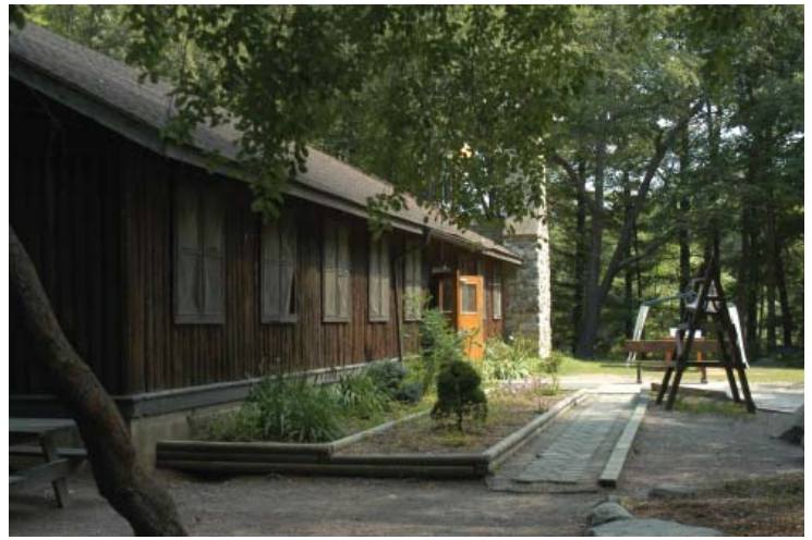
Camp Mason's venerable dining hall awaiting renovation
